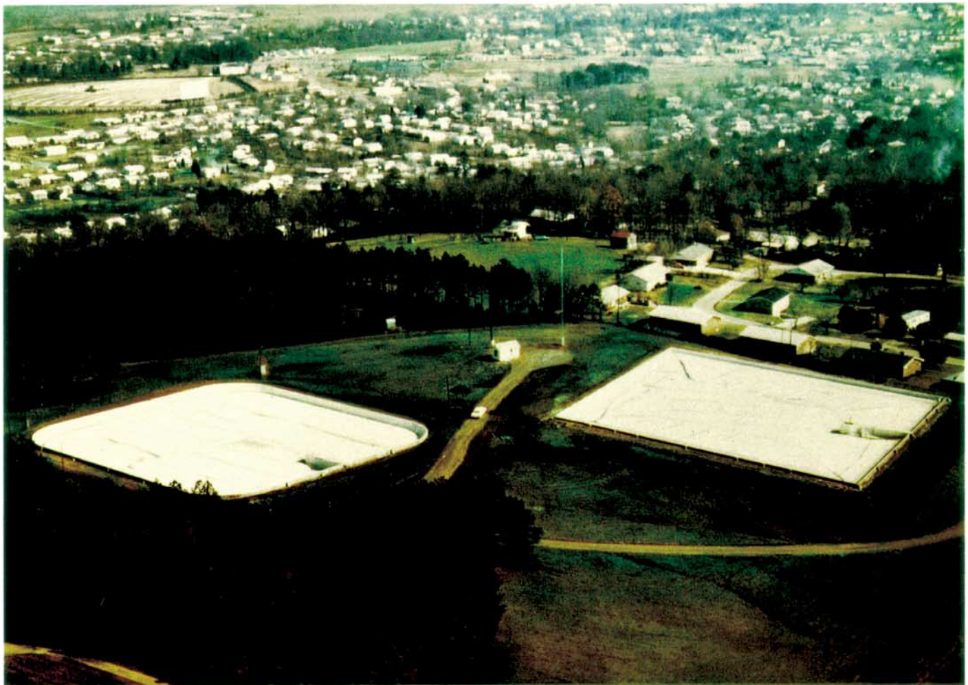
Floating covers: Alcoa, Tennessee, installed 1971
